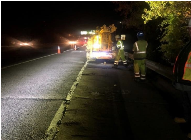
Proposed and as drilled pavement core location
