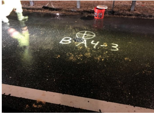
As drilled Pavement Core Location
