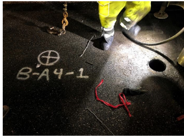
As drilled Pavement Core Location
