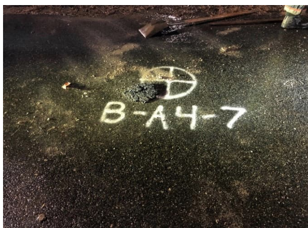
As drilled Pavement Core Location
