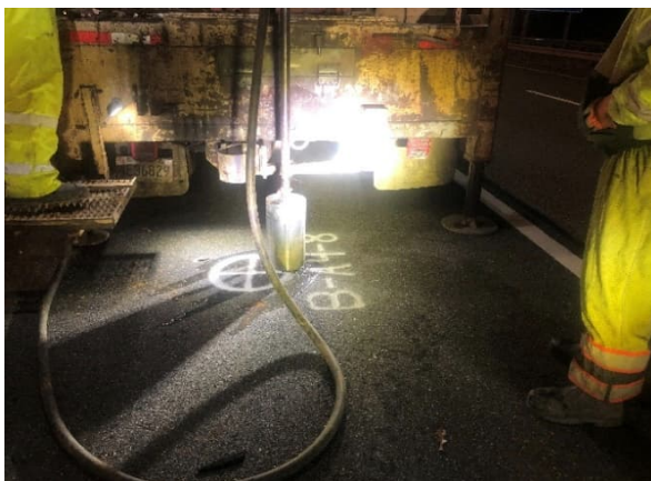
As drilled Pavement Core Location
