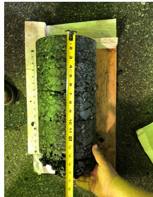
Pavement Core Sample
