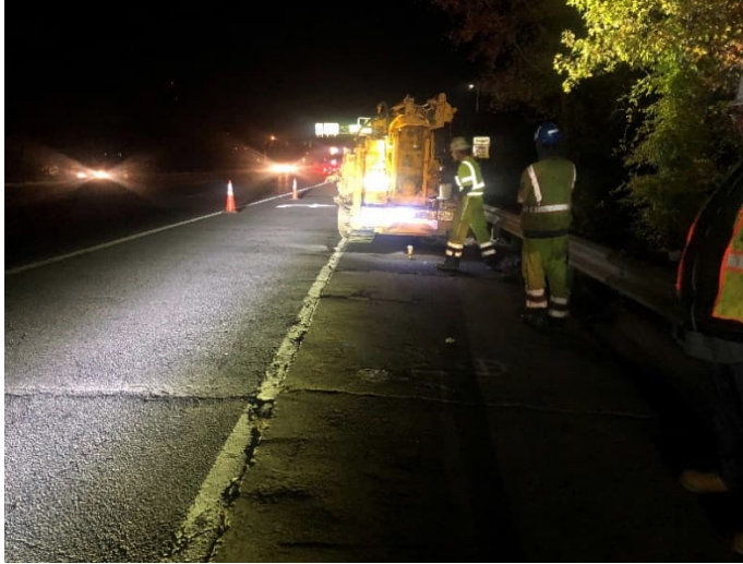
Proposed and as drilled pavement core location
