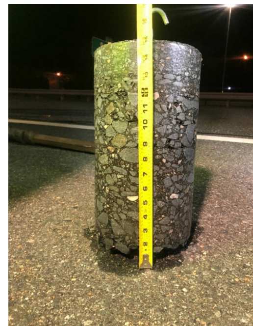
Pavement Core Sample
