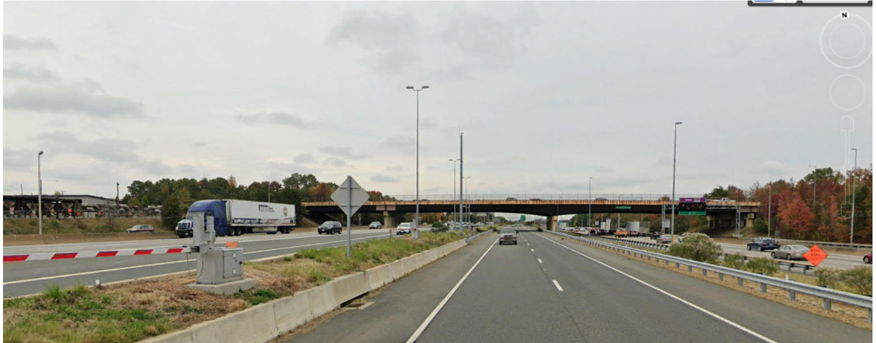
Picture 1: View of Existing Bridge -Looking North, Express Lanes Between Pier-1 and Pier 2 (Photo: Google Earth -Street View)
