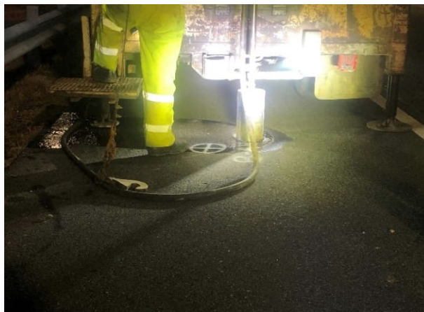
As drilled Pavement Core Location
