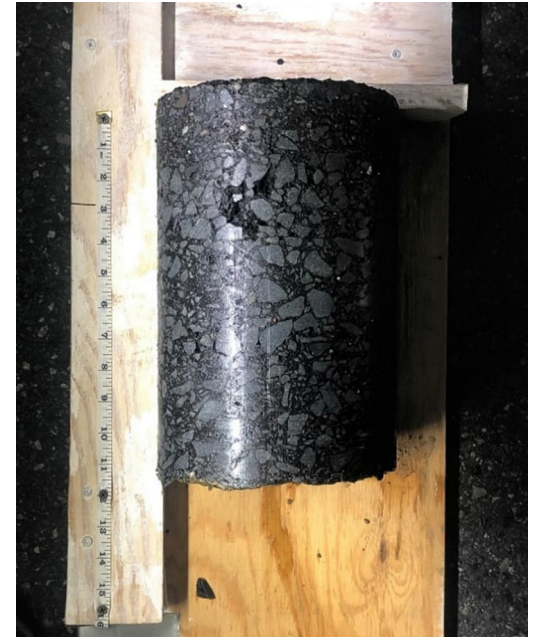
Pavement Core Sample
