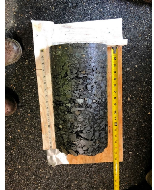
Pavement Core Sample
