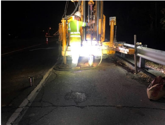
Proposed and as drilled pavement core location
