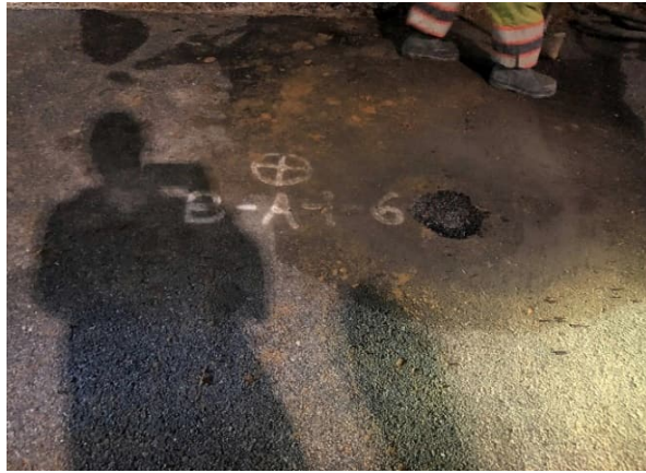
As drilled Pavement Core Location
