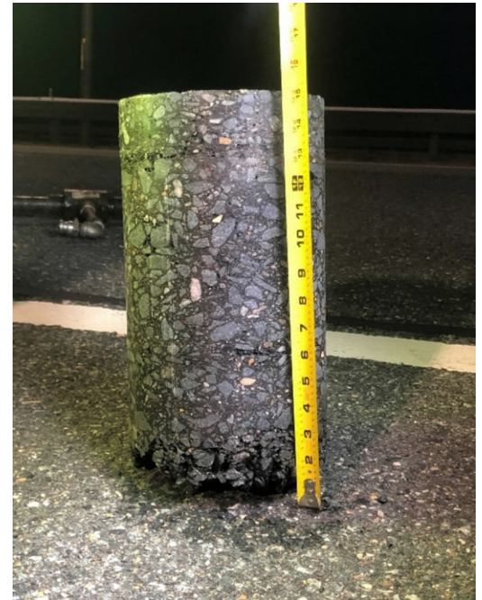
Pavement Core Sample
