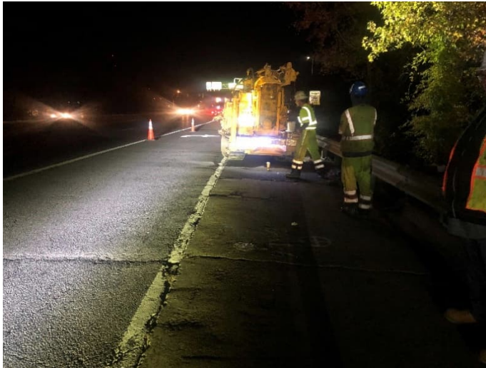
Proposed and as drilled pavement core location
