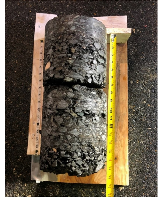
Pavement Core Sample
