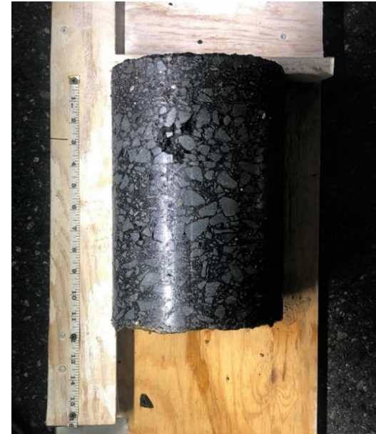
Pavement Core Sample
