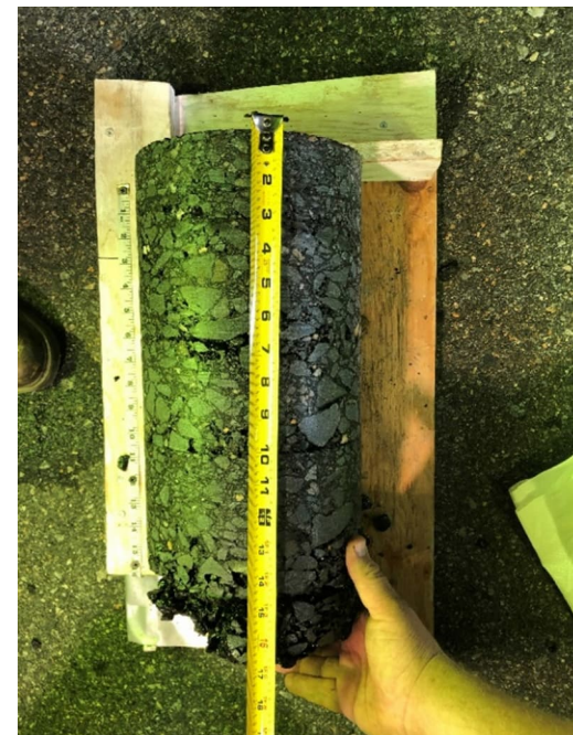
Pavement Core Sample
