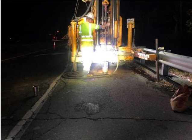
Proposed and as drilled pavement core location
