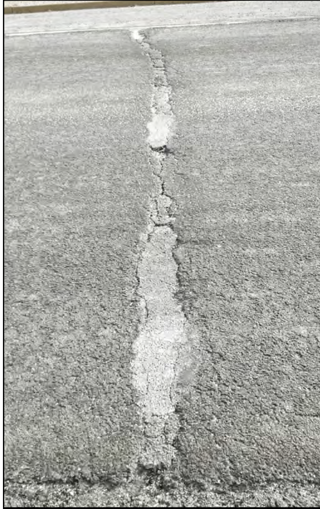
Joint Number: 688 Station: 1691+62 Width: 9'
