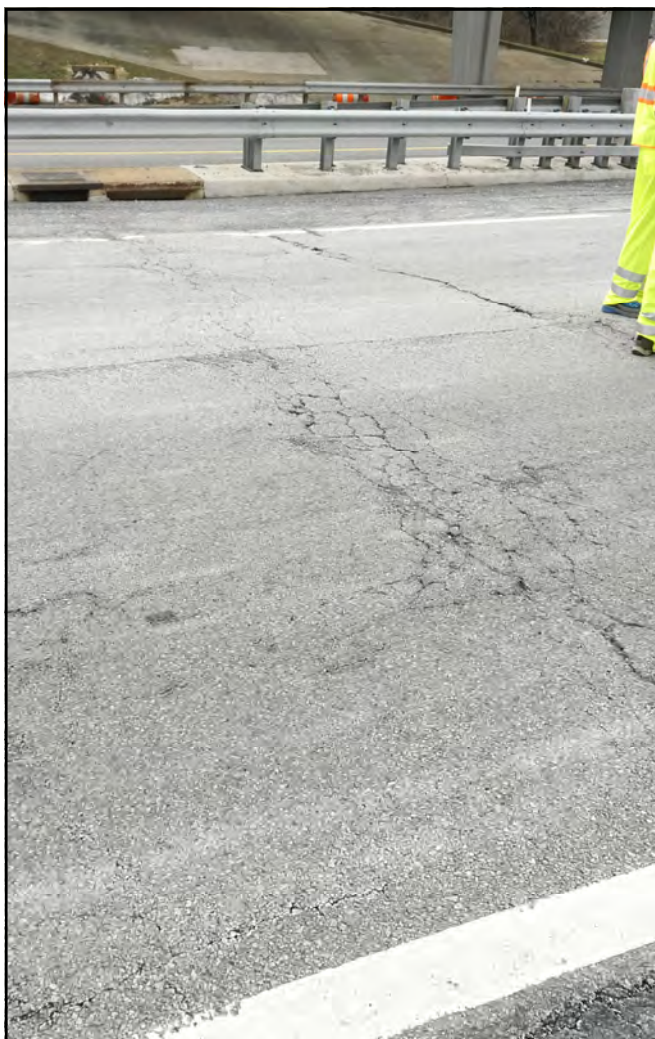
Joint Number: 1005 Station: 1579+35 Width: 19'
