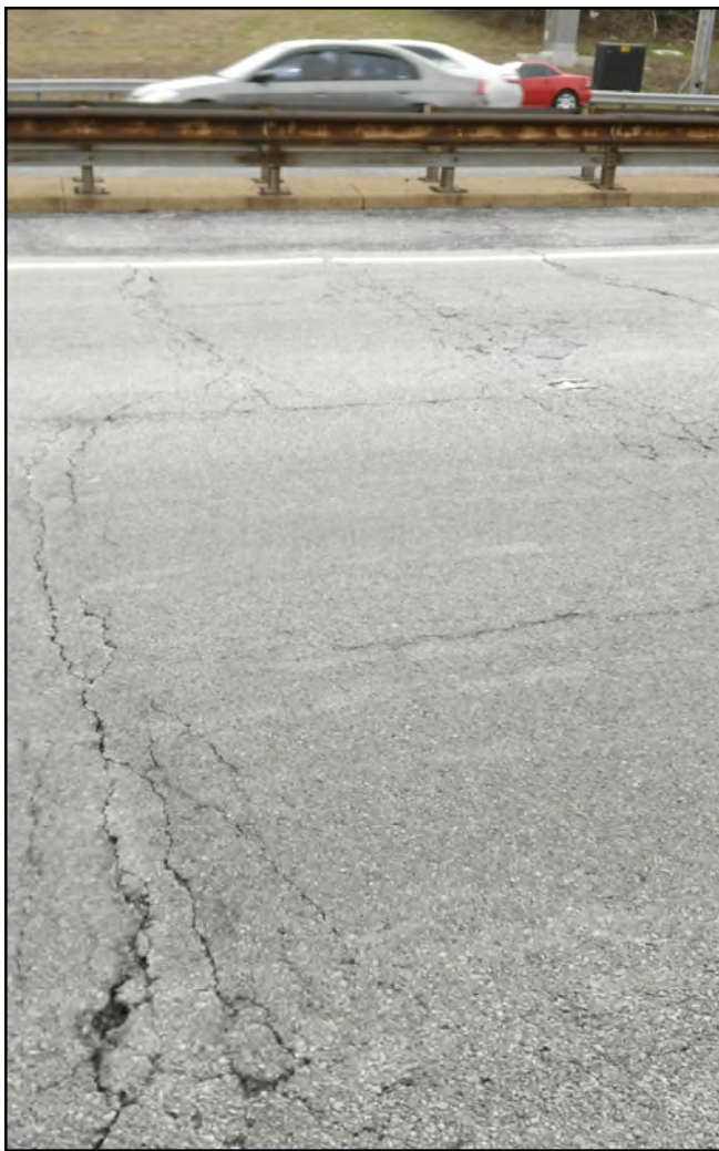
Joint Number: 1007 Station: 1576+62 Width: 18'
