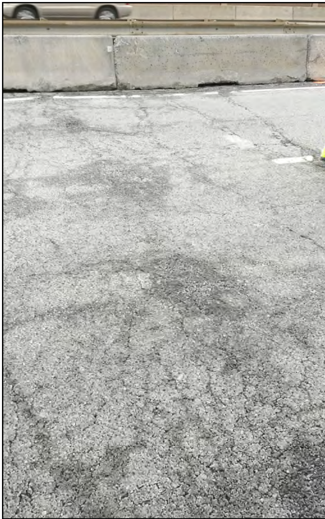
Joint Number: 951 Station: 1613+68 Width: 15'
