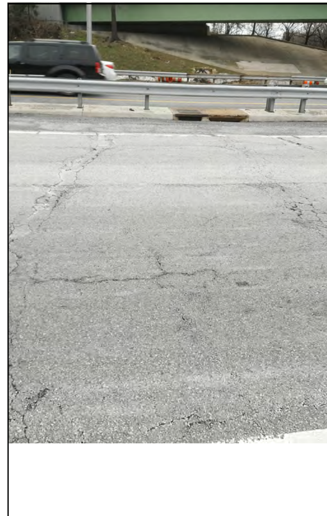
Joint Number: 1005 Station: 1579+35 Width: 19'
